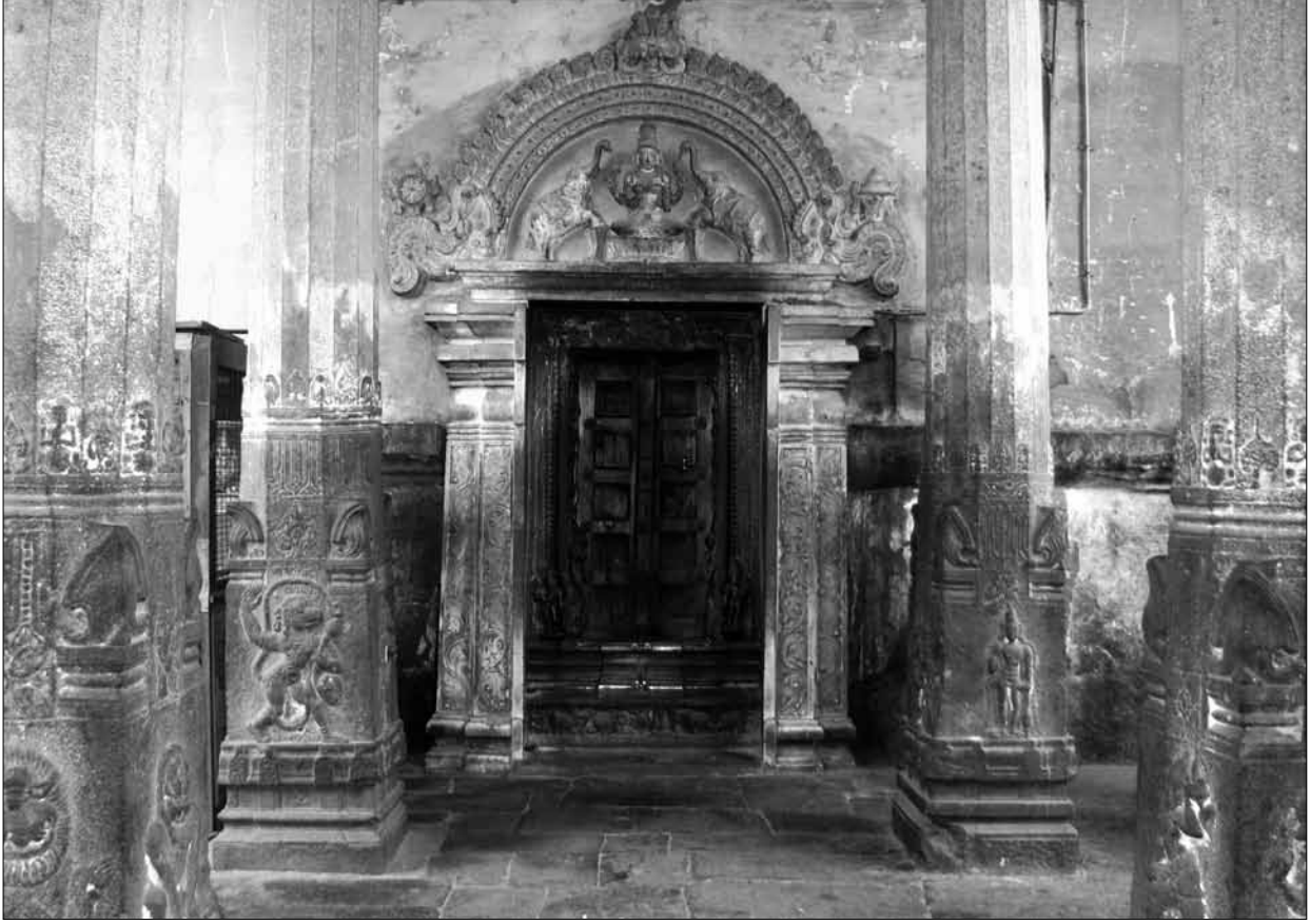
Inner doors to the deity chamber at the Varadaraj temple in Kanchipuram
